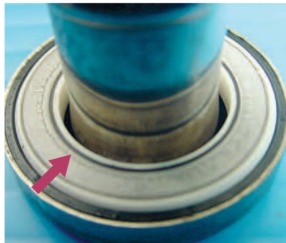
Damaged Accumulated sludge (Contaminated coolant).
